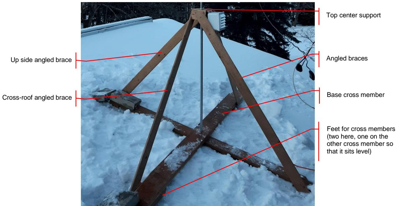
Start by nailing or screwing one of the 1' length feet to each end of a cross member. This will be the bottom cross member in the photo above. Do the same to the other cross member but there are two feet needed on each end so that this top cross member sits level.
